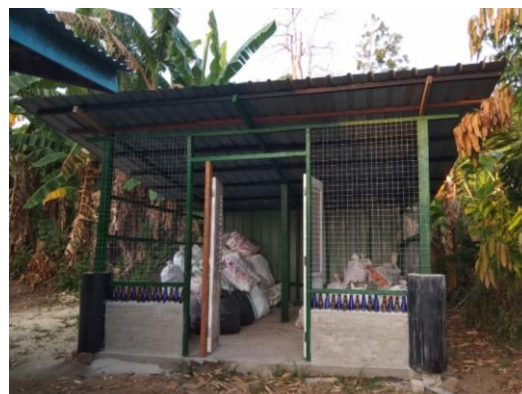
Recycling centre in Kg Air Batang
