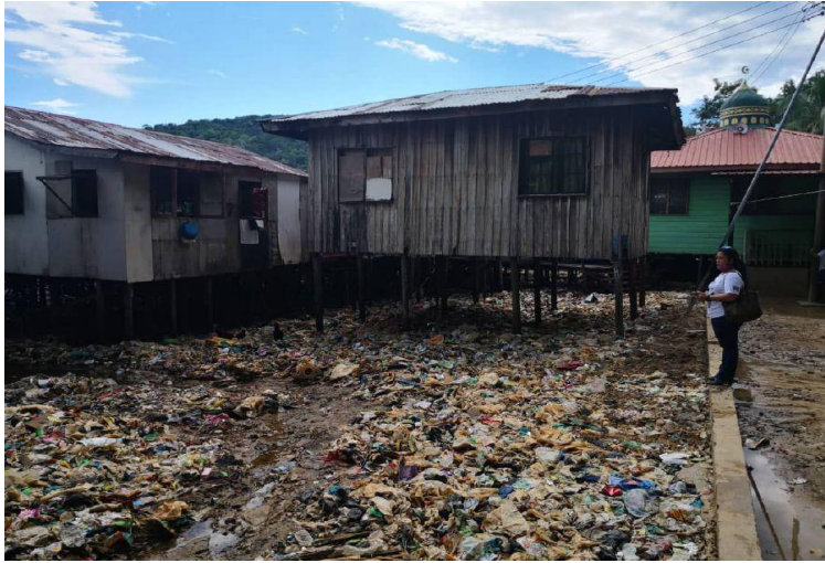
Piles of garbage under the stilt houses of Pulau Gaya (Blu Hope)
